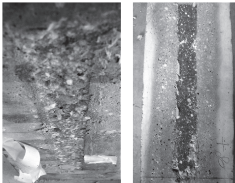
Figure 16 — (a) Failure in the concrete and (b) in the adhesive.
