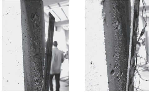
Figure 11 — (a) Failure in the concrete and (b) in the adhesive.
