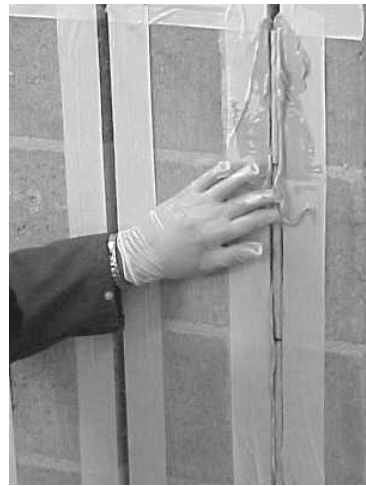
(b) Encapsulation of FRP Bar
