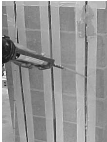
(a) Application of Embedding Paste
