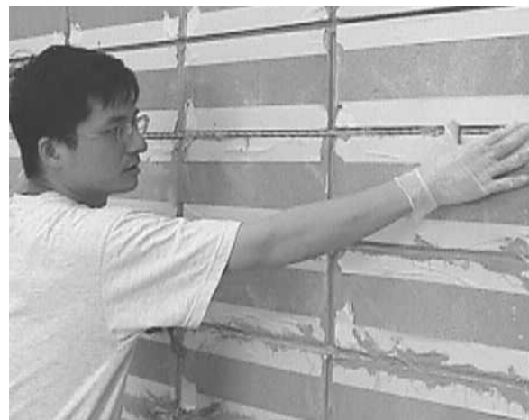
(b) Installation of GFRP Bars
