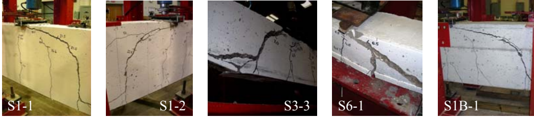
Figure 3. Photographs of failed specimens.
