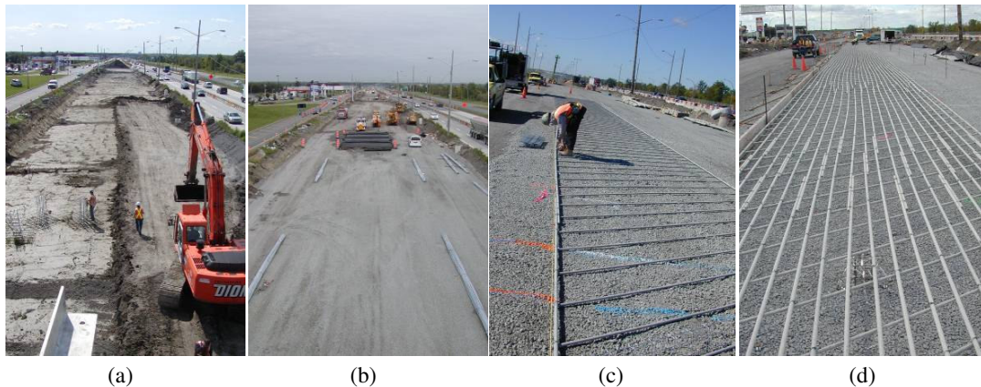
Figure 2. Construction of the test project
