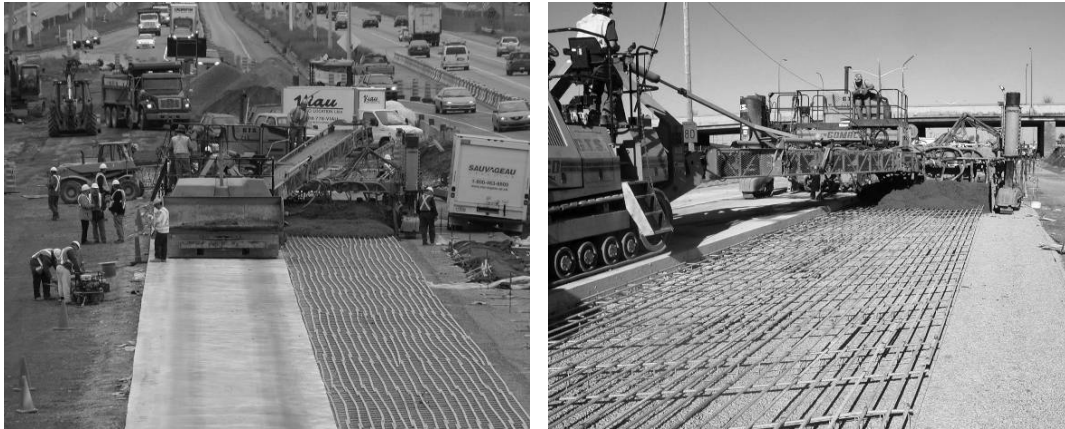
Figure 3. Concrete casting
